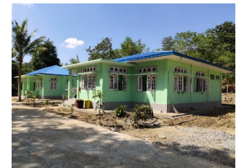
Construction of Rural Health Center
