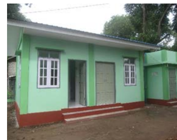
Adding delivery room to Inbatkone Sub-center
