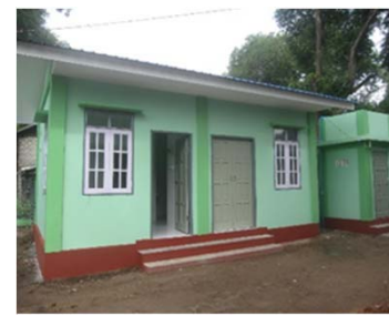
Adding delivery room to Inbatkone Sub-center
