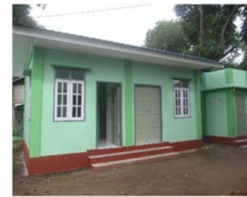
Adding delivery room to Inbatkone Sub-center
