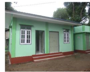
Adding delivery room to Inbatkone Sub-center
