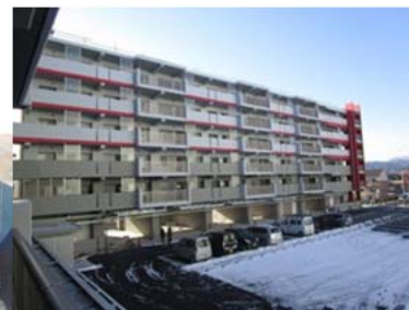
Newly built public housing
