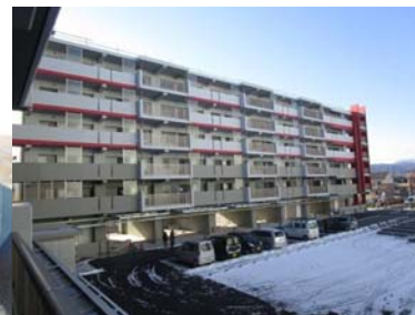
Newly built public housing
