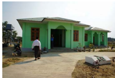
The left building is the clinic, while the right is the midwife's residence.
